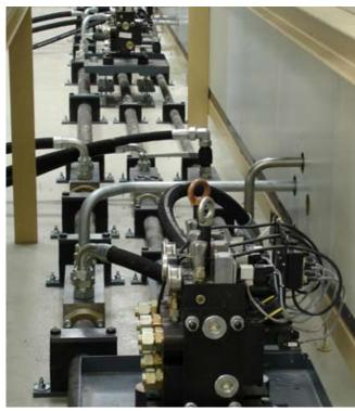
Figure 3: New ring main to expand the central hydraulic oil supply
